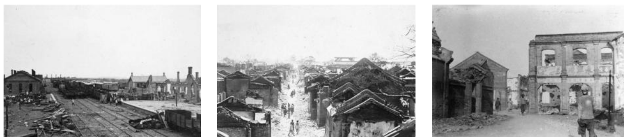
The devastation of Tianjin.
