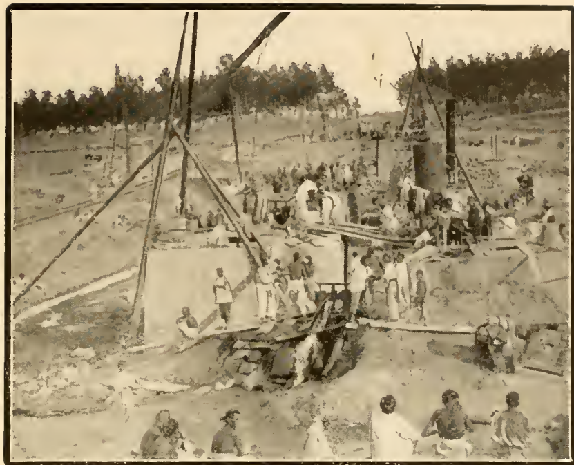
GERMANS BUILDING RAILWAY BRIDGE IN SHANTUNG
