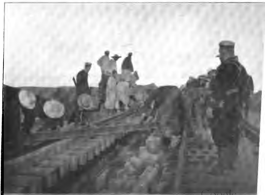
CHARRED SLEEPERS AND WARPED RAILS ON THE LINE OUTSIDE TIENTSIN.
