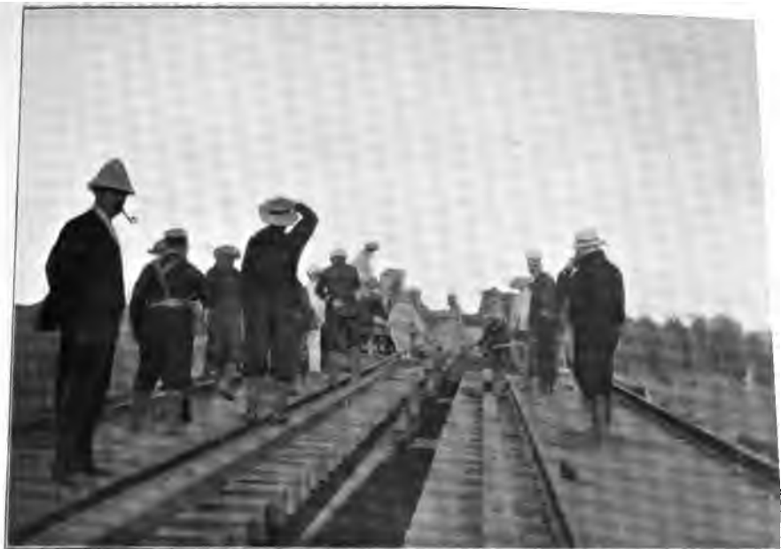
REPAIRING THE LINE OUTSIDE TIENTSIN.
