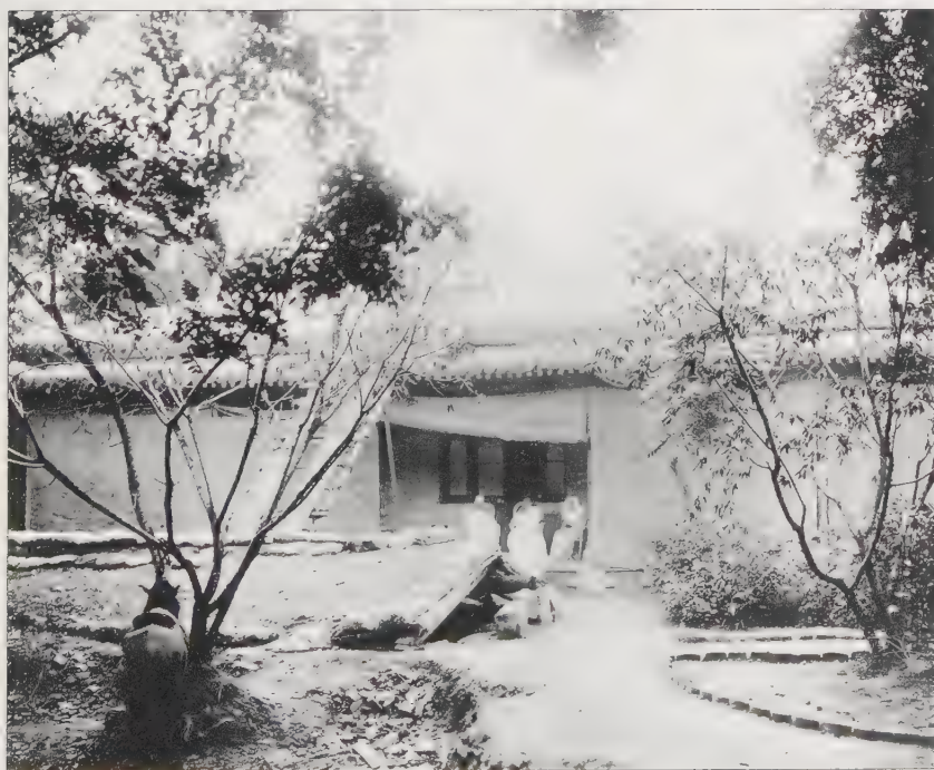
The entrance to a bomb-proof cellar in the British Legation compound is shown in the foreground of this photograph taken by Revd C.A. Killie. In the background can be seen the entrance to the Legation Chancery, which was used during the siege as a hospital. In the entrance sits Matron Lambert seated with two nursing assistants. (Jean S. and Frederic A. Sharf Collection)
