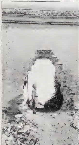
Hole created in the wall of the Imperial City by British Troops as it appeared in a photograph by the Royal Engineers. This hole was very close to the British Legation compound. Two companies of the Royal Welch Fusiliers were sent to hold the Llama Temple in the Forbidden City about half a mile from the British Legation but a hole first had to be made in the south wall to allow access. (Jean S. and Frederic A. Sharf Collection)
