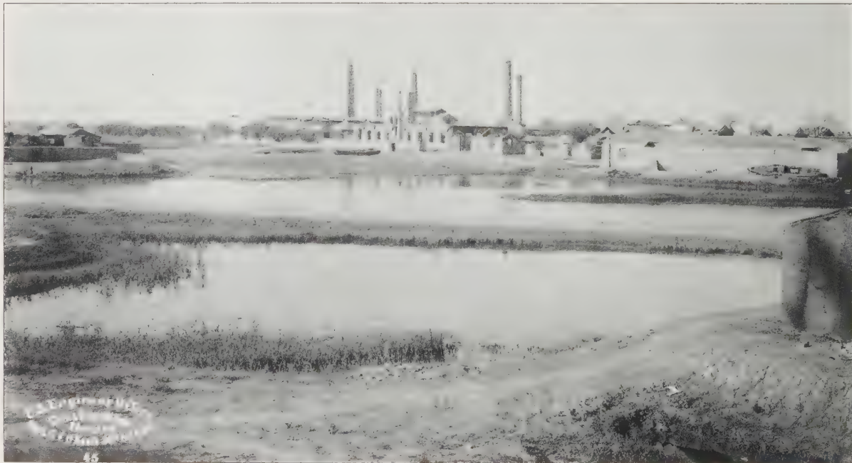
BELOW One of the Chinese arsenals at Tientsin as photographed by C.F. O'Keefe in July 1900 after Tientsin had been relieved. Around Tientsin were the main Chinese arsenals including the ones at Hsiku and Han Yang. The building at Han Yang was the only one not destroyed in the rebellion. (Jean S. and Frederic A. Sharf Collection)
