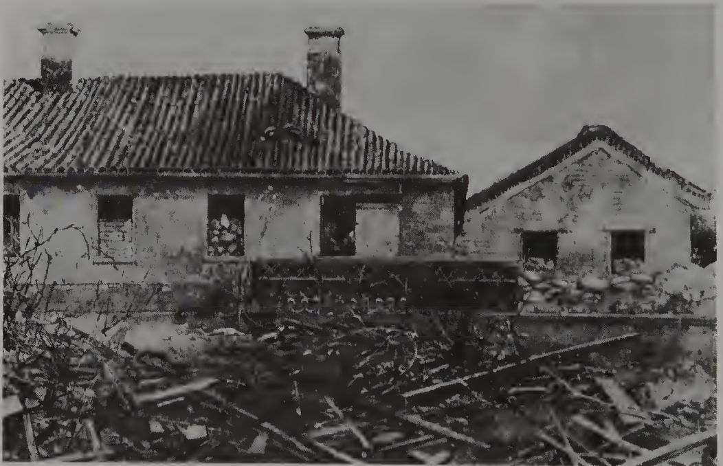
The ruins of the student-interpreters' (fledgling diplomats and customs officials) quarters near the Han-lin. ( Illustrated London News )
