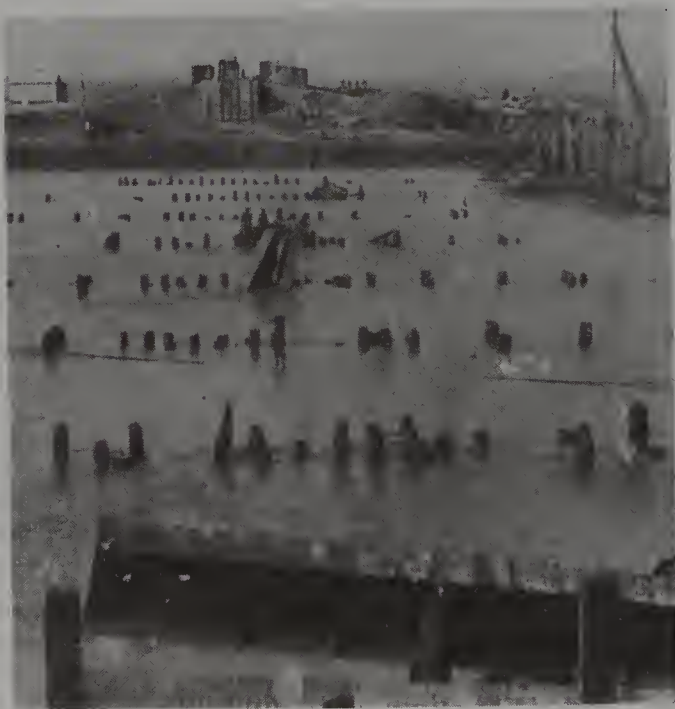
A railway bridge on the Tientsin-Peking line destroyed by Boxers. ( Institution of Royal Engineers )
