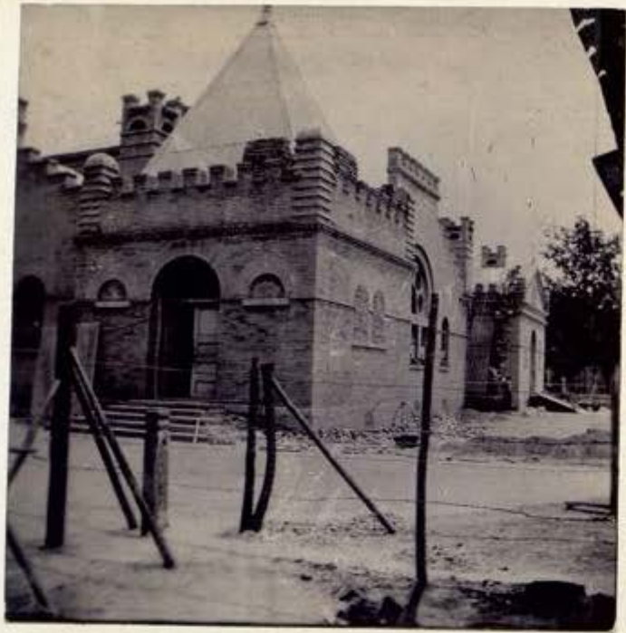
In the Methodist Compound. The Chapel. Some of the windows were bricked up to prevent the enemy from setting fire to the building, and others are loop-holed for rifles.
