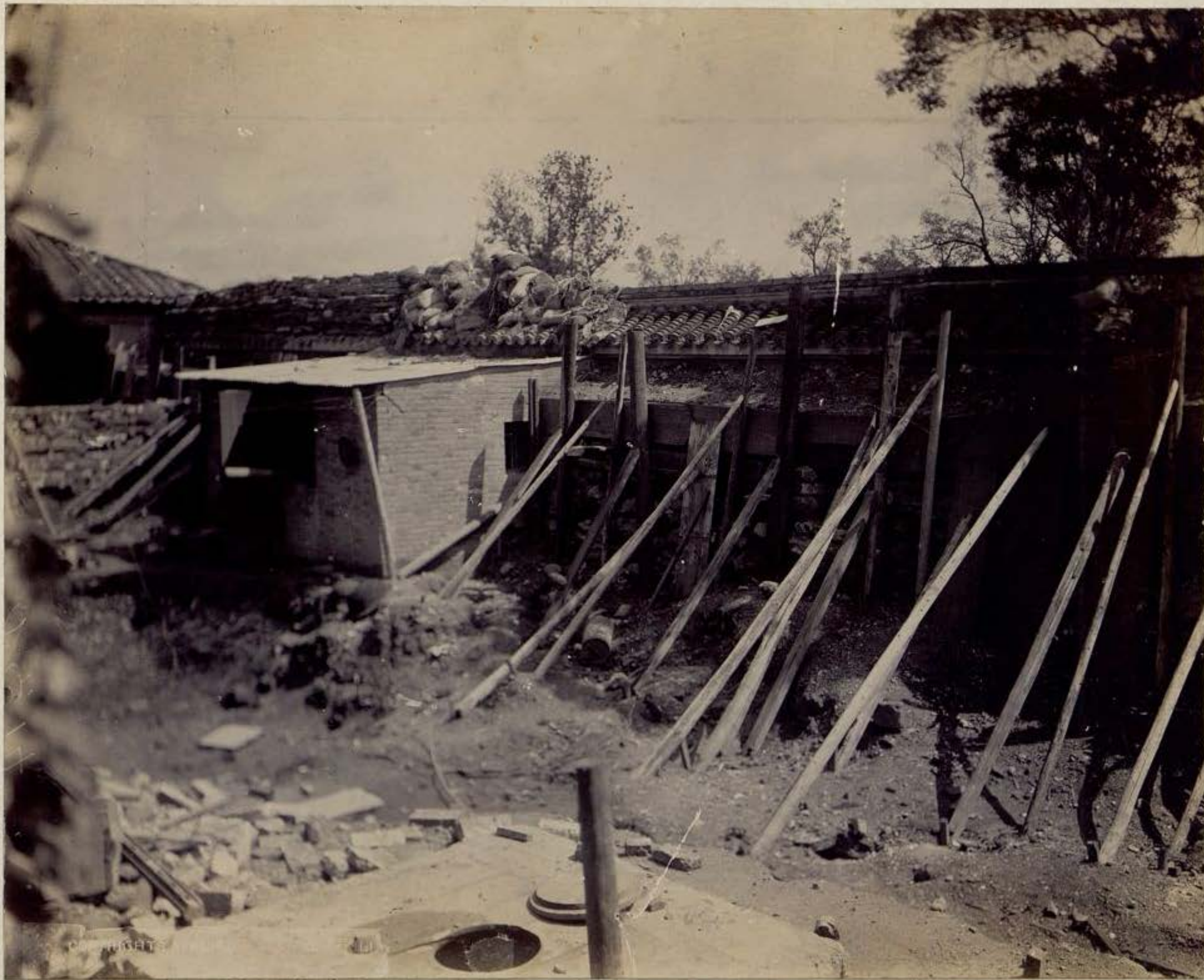
In the British Legation. A section of the outer wall, showing how it was reinforced on the inside with earth, stone, and timbers. When so reinforced, the total thickness was about six or seven feet. No cannon shot ever penetrated one of these fortified walls.
