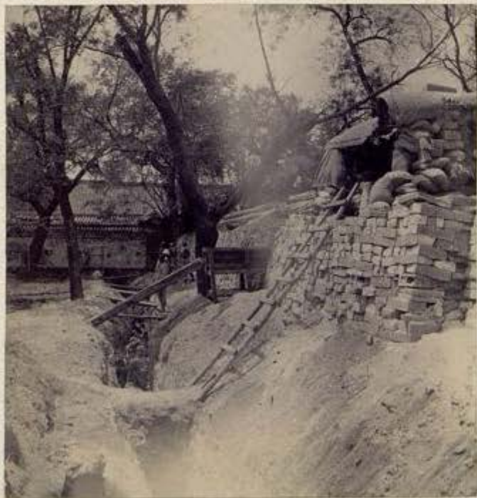
In the Hanlin Yuan. A sentry-post on the outer (Northern) line of fortifications. Native Christians digging countermines. Just this side of the building shown in the picture (in the adjoining court to the West) the enemy was discovered undermining our guard post, and was driven away.
