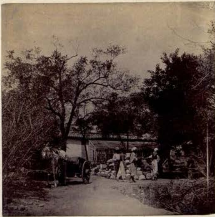
In the British Legation. Hauling the filled sand bags to the places where they were needed. Not less than 50,000 of these bags were made by the ladies, the materials therefor ranging from the coarsest and cheapest, to the finest of silks, satins, and brocades—worth, in some cases, $12.00 per yard, or even more.
