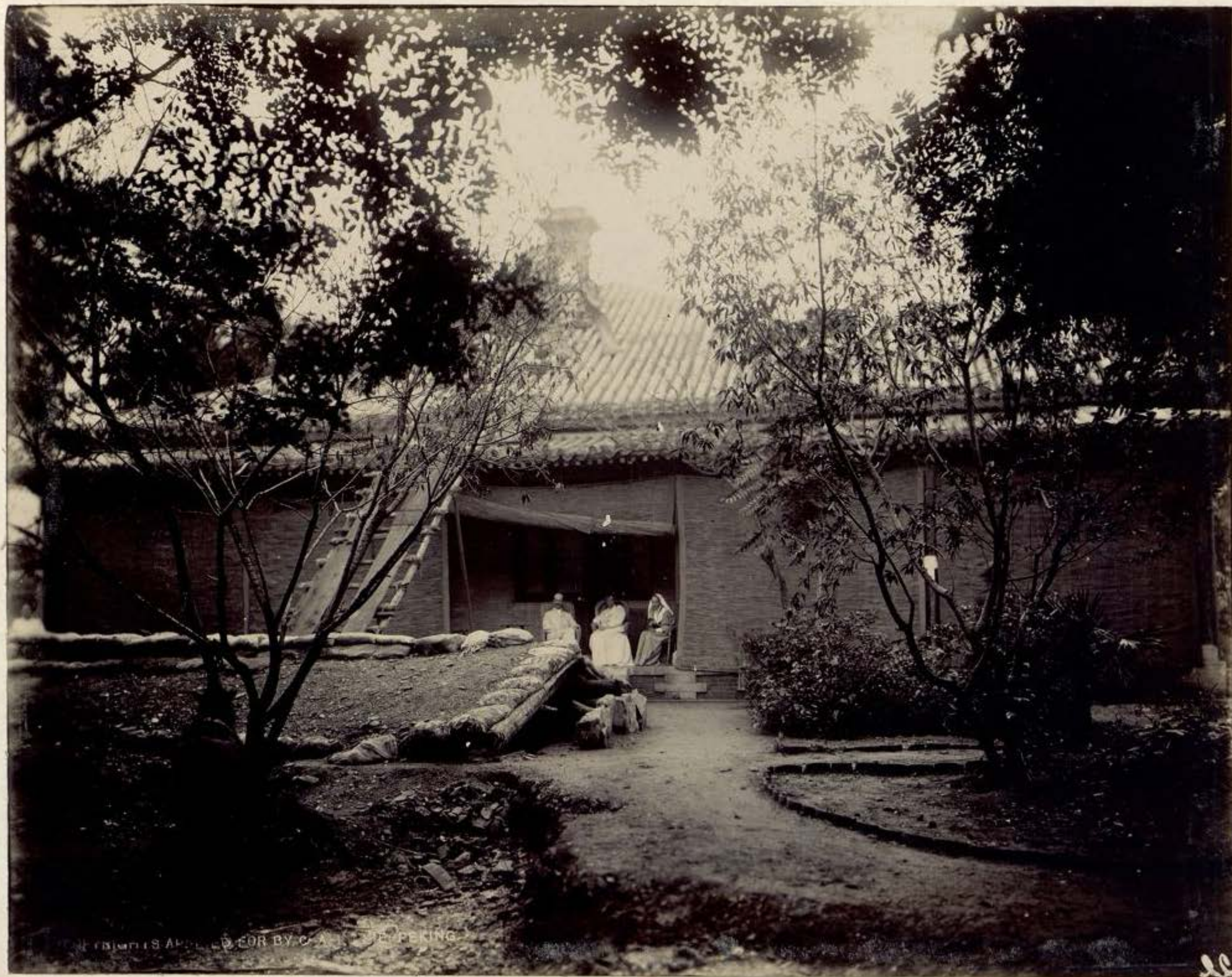
In the British Legation. Secretary Cockburn's House, with a "Bomb-proof," three or four feet deep, in front of it. The earth in the yard was dug up and used to fill sand bags. There was a sentry post on the roof. The inclined way was prepared for the purpose of taking a rapid-fire gun up on to the roof.
