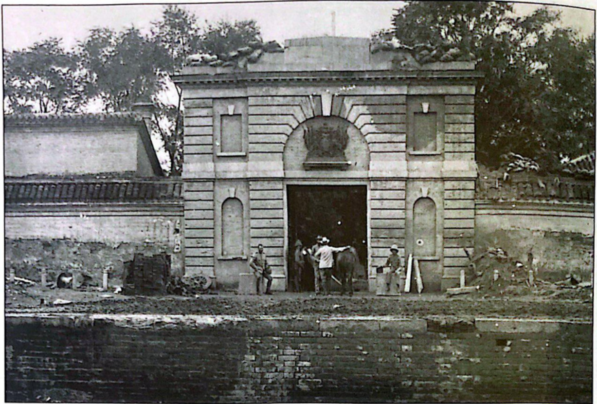
The entrance to the British Legation compound after the siege. The barricade has been removed. The canal runs in the foreground. Photograph: Royal Engineers.
