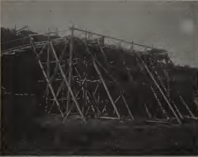
ABOVE: Repairing a sabotaged railroad (National Army Museum)
