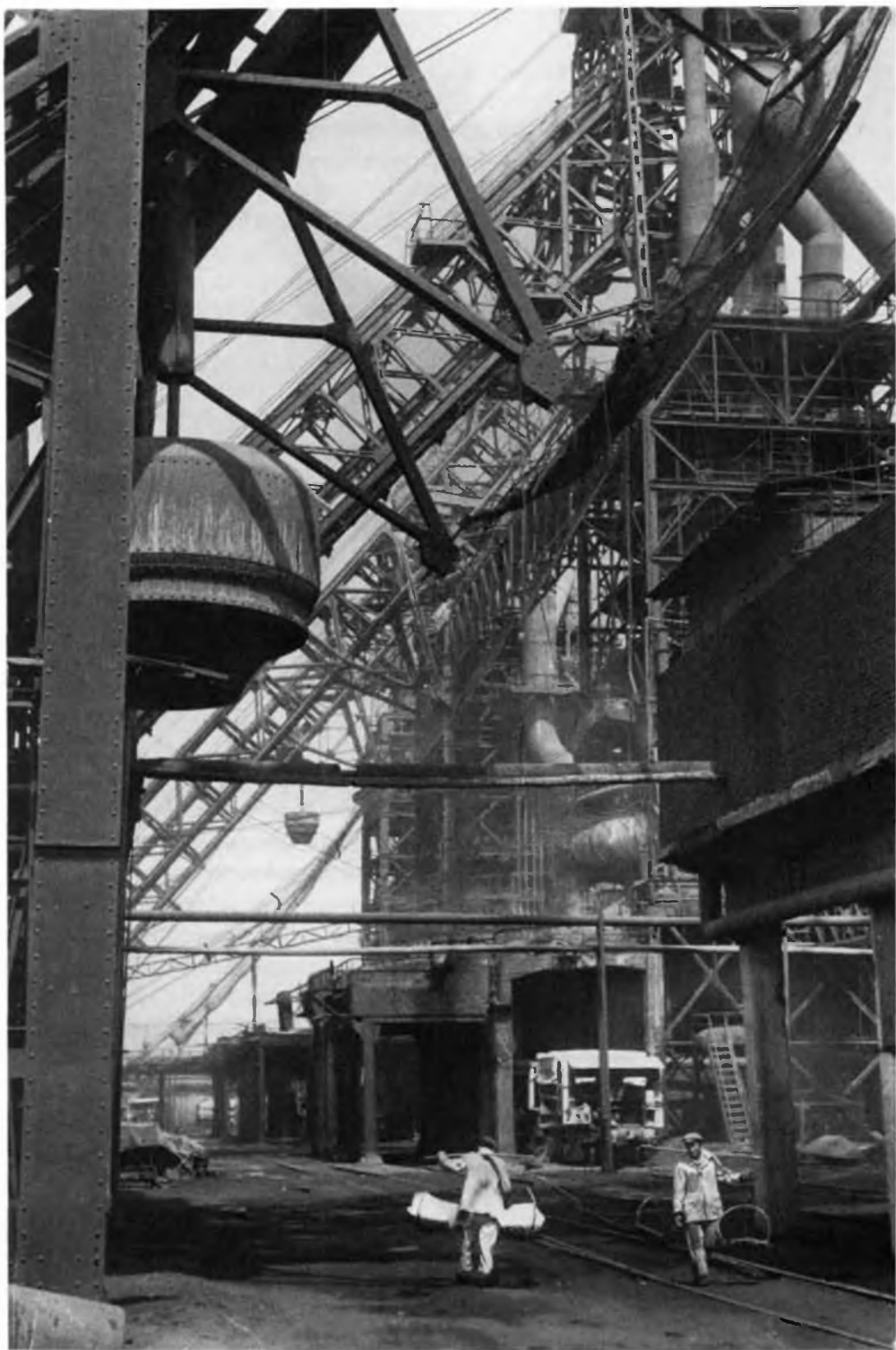
Steel mill, Anshan, Manchuria, 1958 (photograph by Henri Cartier-Bresson)
