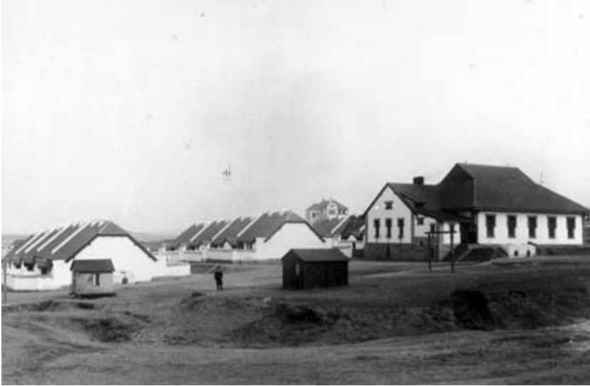
FIGURE 7.7 Housing for Chinese apprentices in Qingdao (German colonial period). From BA-MA-Freiburg, Nachlass Truppel, vol. 62, p. 11, verso.
