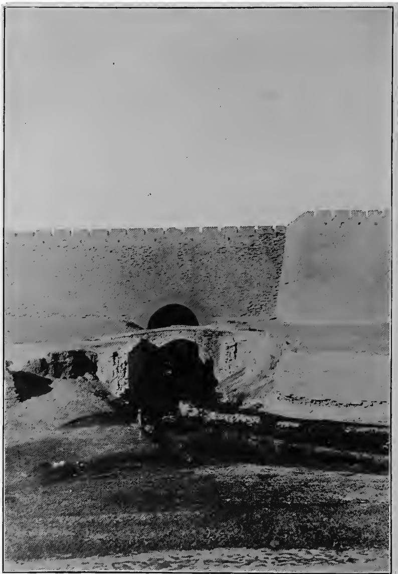
SLUICE GATE WHERE THE BRITISH ENTERED.
