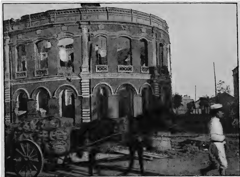
RAILWAY ADMINISTRATION BUILDING, TIENTSIN, SHOWING EFFECT OF SHELL FIRE.
